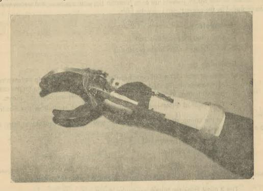
The forearm and palmar portion are attached on to the stump by velcro straps.
